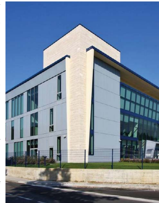
CNAO facility in Pavia, Italy
